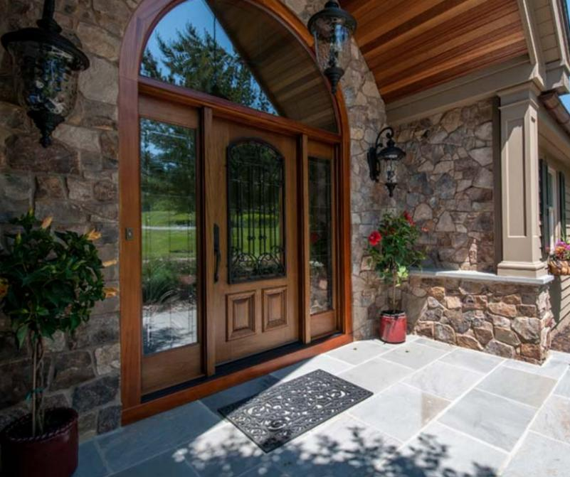
The below entrance makeover incorporated a new roof pitch, low-maintenance composite columns and fascia, stone facade, a flagstone porch and steps as well as a cedar porch ceiling. The impressive mahogany front door and windows are decorated with wrought iron accents that are complemented by the matching chandelier and porch lights. Note the wide flagstone steps that provide ample room for accessorizing with colorful planters or seasonal decorations.
