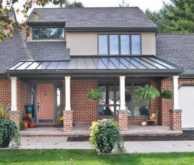
The above porch facelift incorporated a metal roof to match the contemporary look of the home. Brick columns were added to match the home's existing brick while the color coordination of the garage doors, columns and stucco adds continuity.
