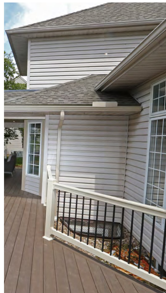
As mentioned on the previous spread, the addition of four basement bedrooms were made possible by installing window wells (one pictured above behind the railing) as a means of egress in each bedroom.
