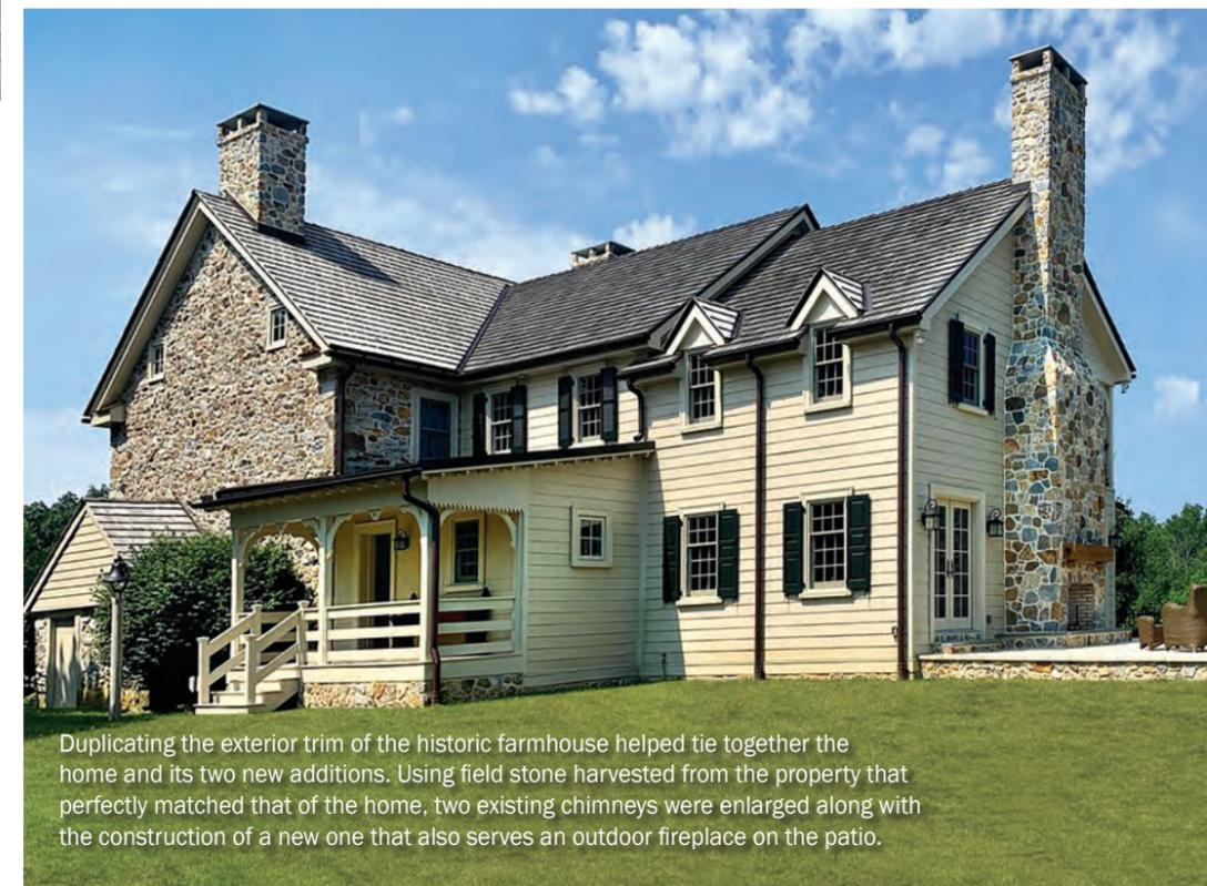
Duplicating the exterior trim of the historic farmhouse helped tie together the home and its two new additions. Using field stone harvested from the property that perfectly matched that of the home, two existing chimneys were enlarged along with the construction of a new one that also serves an outdoor fireplace on the patio.
