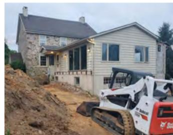
In preparation for the new addition, an unsightly 1960's ranch-style addition attached to the farmhouse was removed down to the foundation. The square footage of the new addition remained the same with the exception of additional space for the dining bay and foyer. With the slope of the yard, it took 56 tri-axle truckloads of backfill to level the property.
