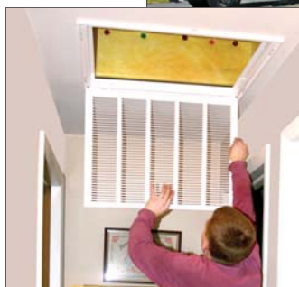
Above is a typical ranch style home without existing air conditioning or duct system. Left, a filter grille is being installed in a hallway for the central return. Filter grilles allow easy filter changes without needing to go into the attic.
