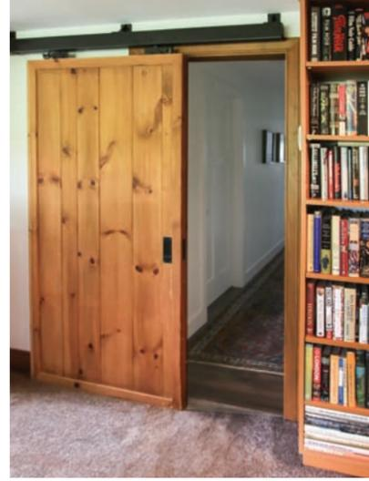
Providing privacy to the master suite, (and fitting perfectly with the rustic atmosphere of the office), is this re-purposed, tongue and groove paneled pine pocket door.
