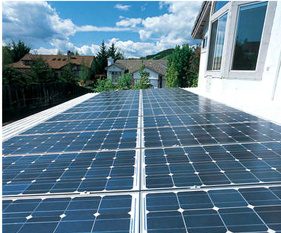
A well-designed PV system needs clear and unobstructed access to the sun's rays for most or all of the day, throughout the year. Usually, the best location for a PV system in the U.S. is a south-facing roof.
