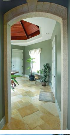
The new garage is connected to the original garage space by a 16' wide octagon foyer which is constructed with an octagon framed cathedral ceiling (19' at its height). As seen in these photos, the ceiling is finished with mahogany tongue and groove boards and 3x6" beams in each corner.
