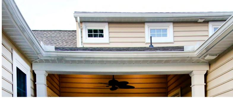
The enlargement of this 2nd floor bedroom was made possible by extending the width of the dormer of the original 2nd floor bath as seen in the BEFORE photo on the left page. Previously, the sloped roof line on the back wall would not have accommodated a bed (let alone one with a headboard).
