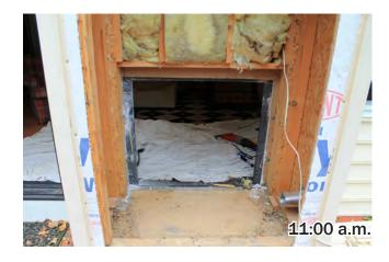
To access the fireplace in this vinyl sided home, we simply opened up the exterior wall. After removal of the old fireplace unit, we installed the replacement unit which was identical in size.
